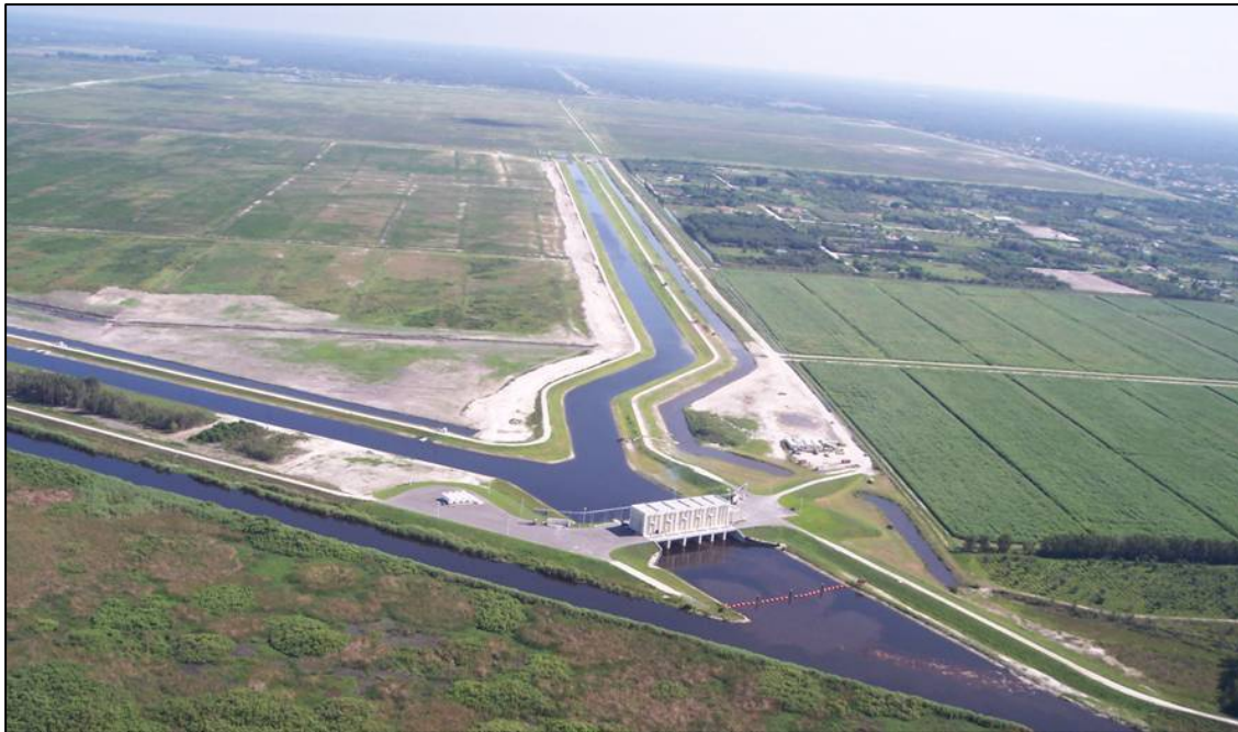
Figure 3-4. Aerial photo of STA-1E prior to substantial completion.
