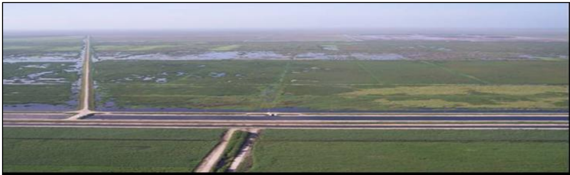
Figure 6-4. Aerial view of Cell 2A looking south from the north levee.
