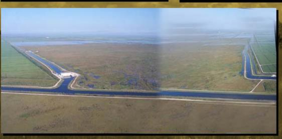
> Stormwater Treatment Area 3/4 is the world's largest constructed wetland! Over 16,500 acres of former agricultural land has been converted to a biological treatment system designed to remove over 55 tons per year of phosphorus from water entering the Everglades.
