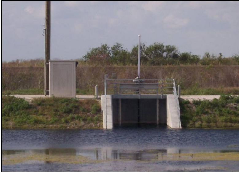
Figure 7. Typical STA-1E Inflow/Interior/Outflow Structure.
