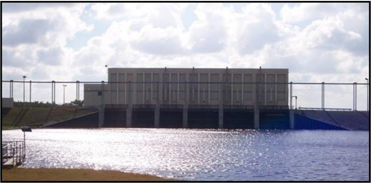
Figure 8. Pump Station S-362.
