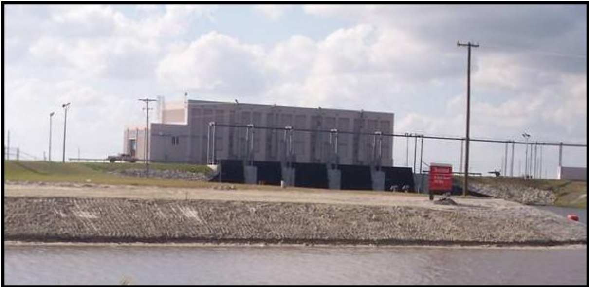
Figure 4. Pump Station S-319 With Western C-51 Canal in Foreground.
