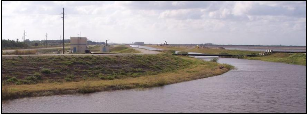
Figure 5. Pump Station S-361.
